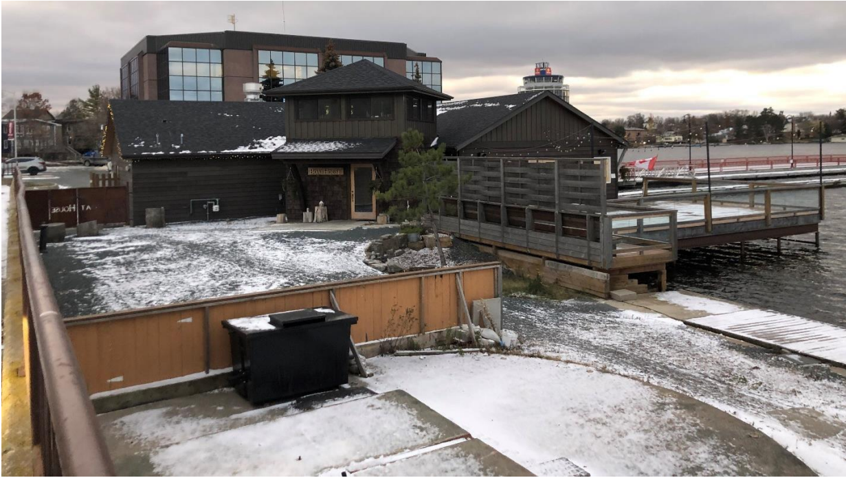
Photo 3 – View of the building from the interior side yard, showing the retaining wall on the left
