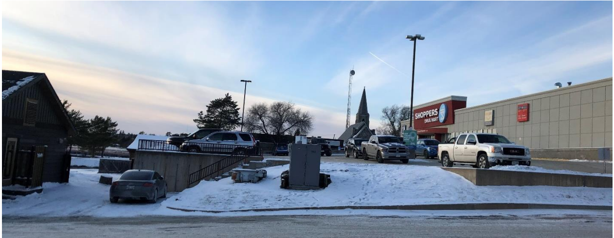
Photo 5 – View of the retained lands, retaining wall, parking lot and Shopper’s Drug Mart
